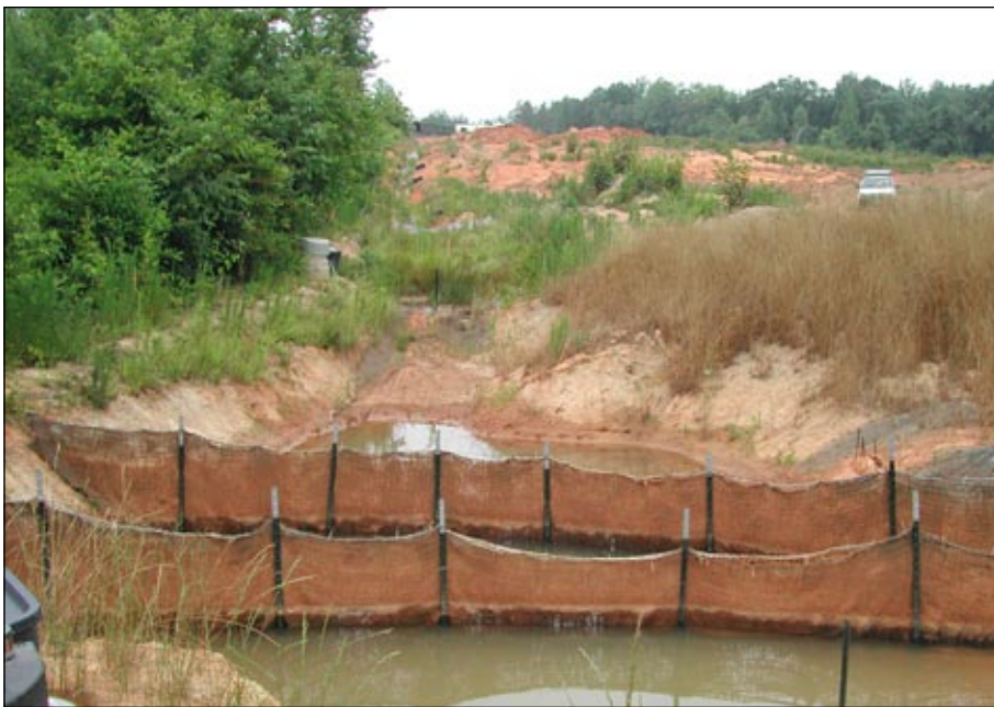
Figure 8. Example of porous baffles made of jute netting backed by coir erosion blanket, as viewed from the outlet.
